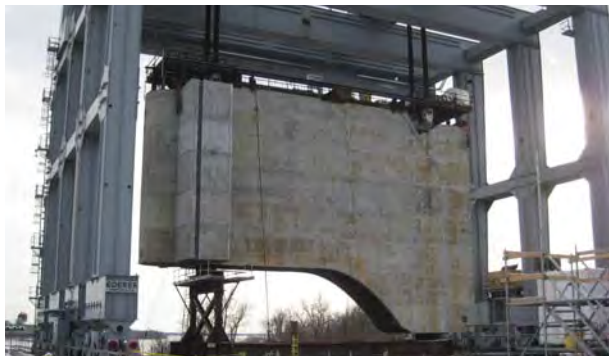
Pier Shell Lift
