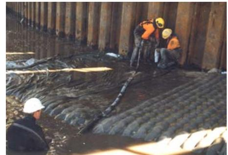
Washout from currents or vessel actions is prevented whilst setting. This creates reliable protection in comparison to grouted rock or tremi concrete.
