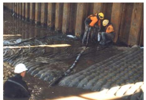
The system is lightweight (0.7 kg/m<sup>2</sup>) for handling and transportation and can be used by contractors and divers worldwide. Proserve undertake scour apron design using appropriate design guides and proven performance. We engineer and fabricate mattress systems to suit site conditions and provide engineering support for installation worldwide .
