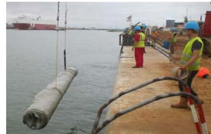
The lower construction thickness of concrete mattress provided a cost effective solution and importantly minimised the span height of the quay wall and maximised its protected embedment depth.
