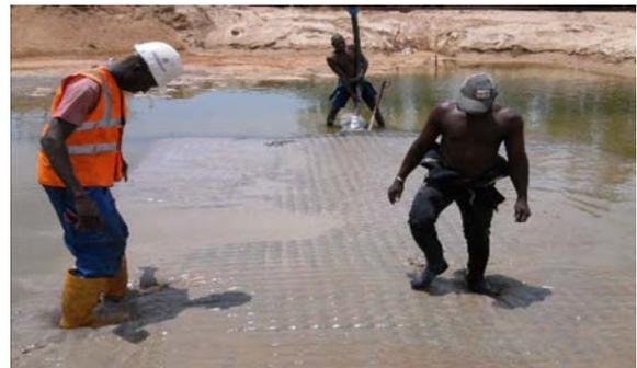
A rip rap stone falling apron edge detail was provided to resist edge scour in the sand and clay bed.
