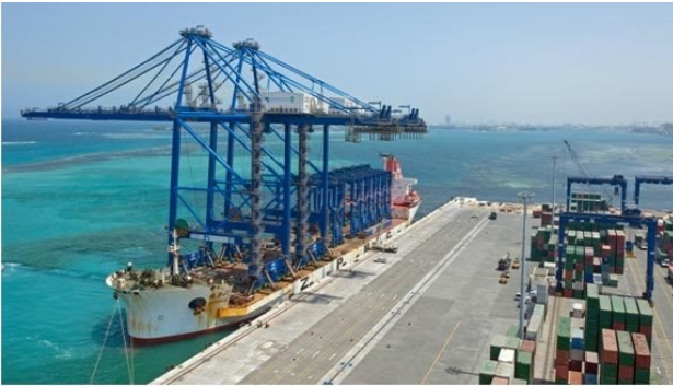
New Quay Extension - Installing Cranes
