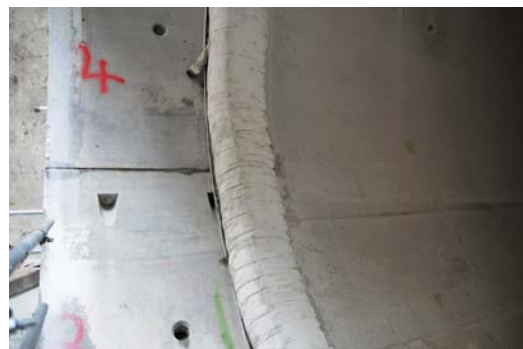
Insitu Concrete Lining Stopend Ringseal
