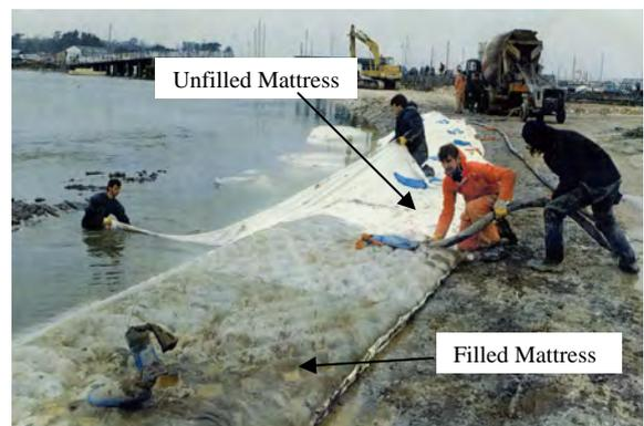
The mattress is then filled by pumping micro-concrete through filler sleeves which are integral to the mattress, uniformly and at the correct rate. Filling is controlled to ensure each panel is completely filled and the fluid head does not exceed 2 m. A job specific Installation Guide is produced for each project. Engineers assistance on site is available.
