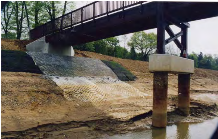
Sewage Works Access Bridge
