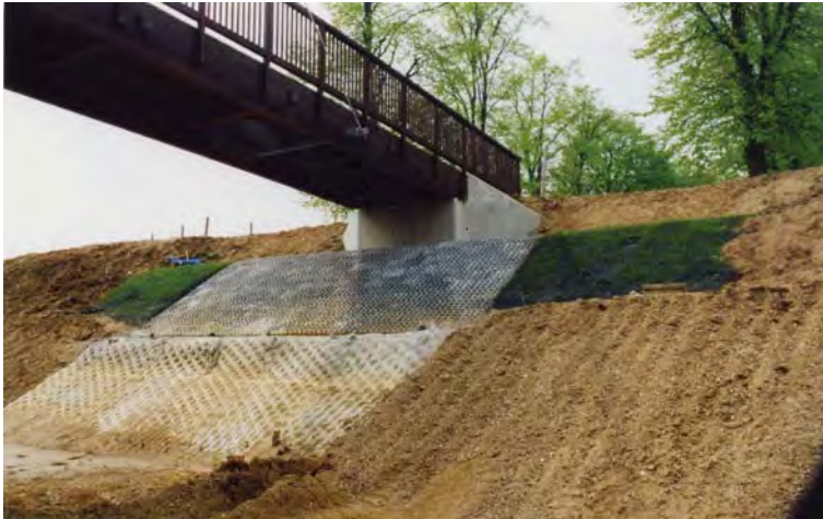
Myrke Footbridge Revetment
