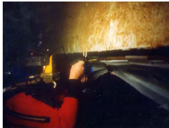
Diver Fixing Mattress to Underside of Tunnel
