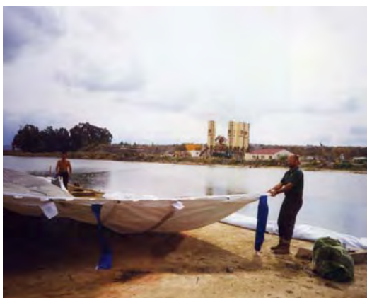
Installation Preparation by Divers
