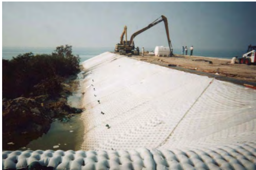
Laid & Filled Mattress Along Embankment
