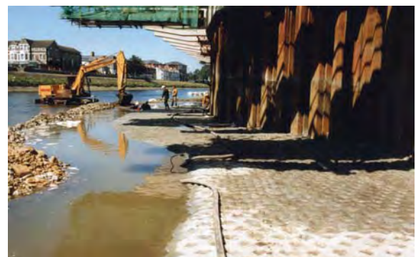
Laid Mattress and Bed Profiling
