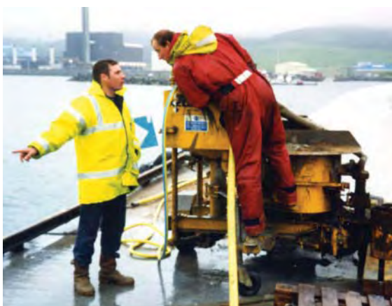
Micro Concrete Mixing and Pumping
