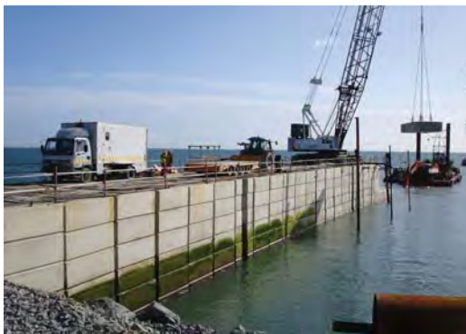
Placing of the stacked blocks
