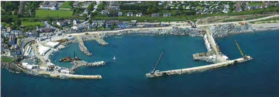
Greystones Harbour during construction
