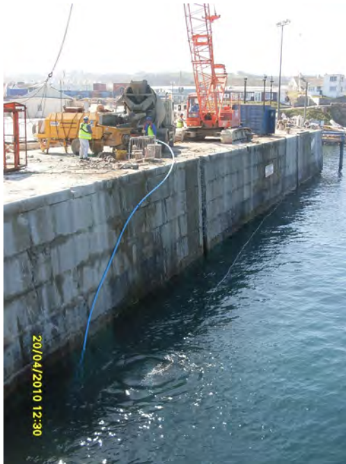
Mattress filling from Commercial Quay
