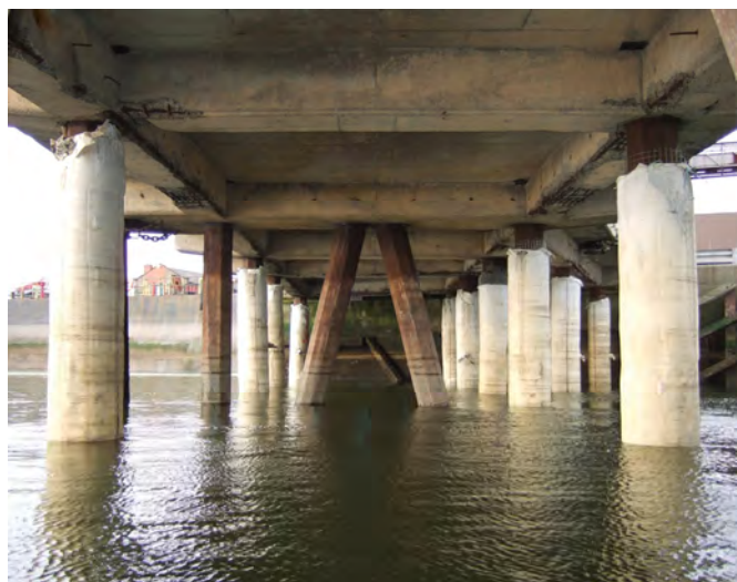
Repaired Piles Using Pile Jackets
