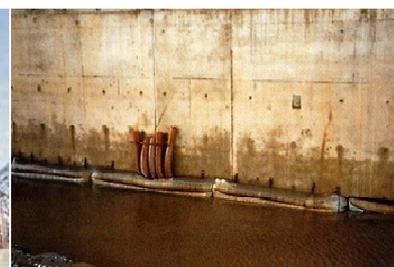
Figure 18 – Grout Bag Foundations
