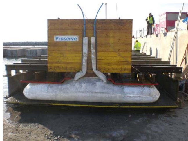
Grout Bag Testing
