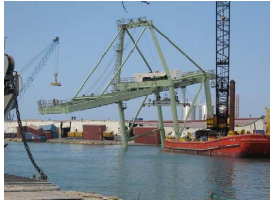
Earthquake Damaged Crane and Jetty
