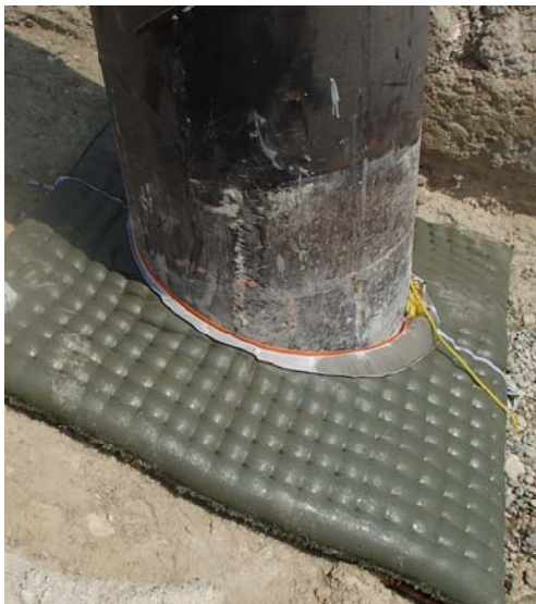
Pile Seal Test
