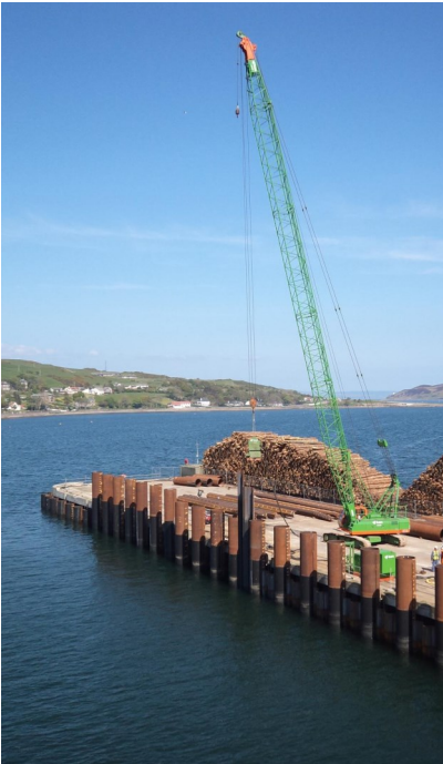
New Combi Piled Quay Wall
