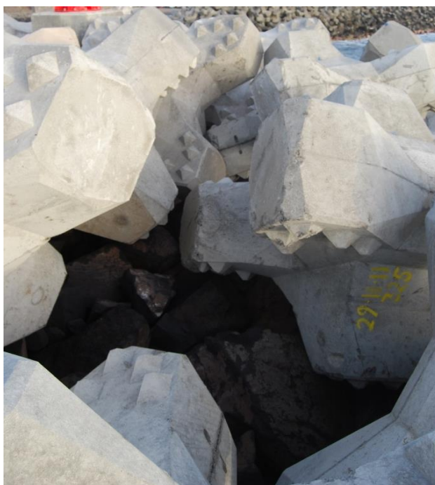
Void between Accropode II units
