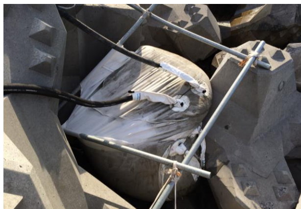
Grout Bag Held in Position
