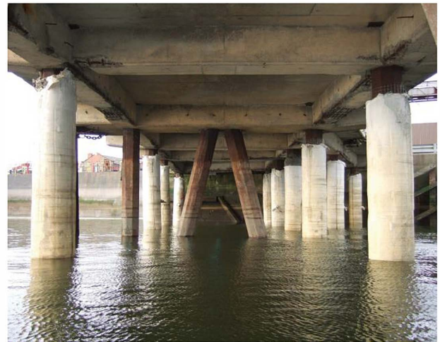
Repaired Piles Using Pile
