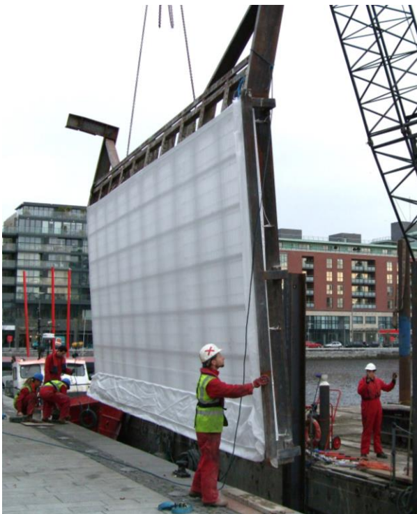
Control Frame Being Craned into Position
