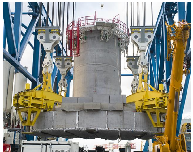
Pier Base (Viaduct Littoral/Sébastien Marchal)
