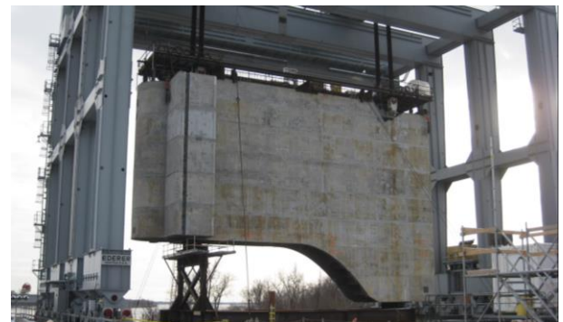
Pier Shell Lift
