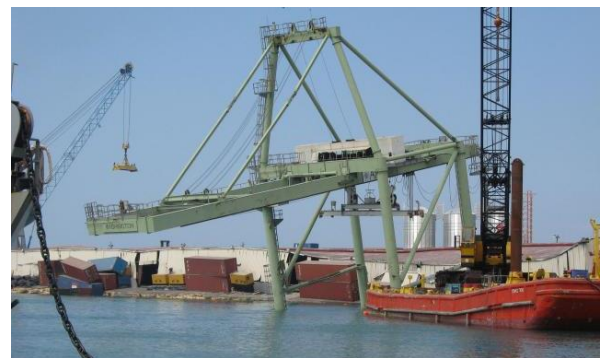
Earthquake Damaged Crane and Jetty
