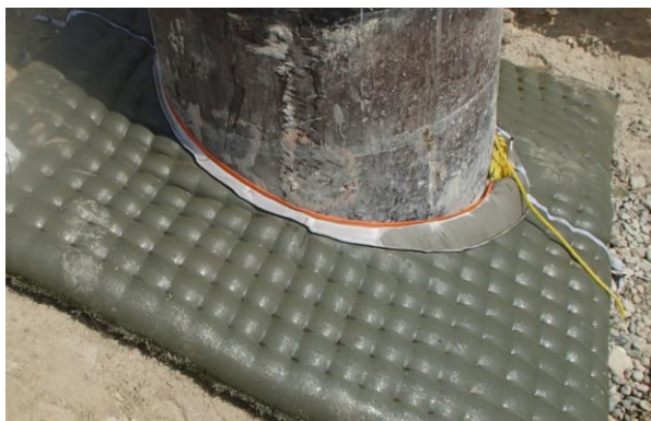
Pile Seal Test
