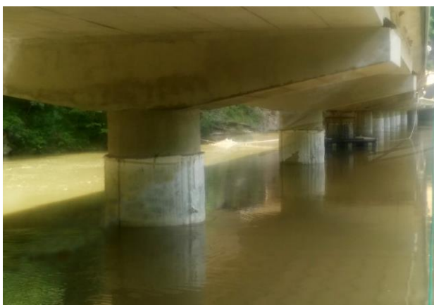
Reinforced Concrete Piles
