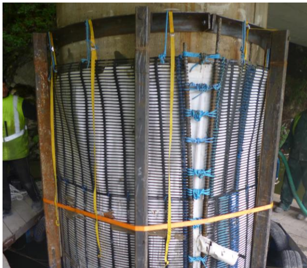
Pile Jacket System with Temporary Steel Frame
