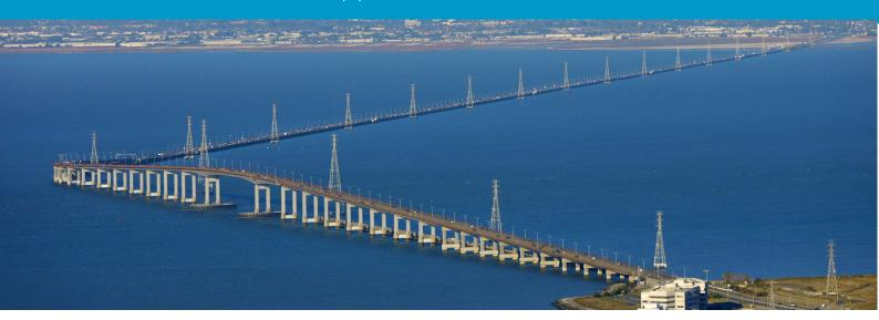
The San Mateo—Hayward Bridge across San Francisco Bay is a 11.3 km long structure. It consists of three sections a 0.1 km approach, a 3.2 km main span across the shipping channel and a 8.1 km trestle structure that ties it to the east bank. In 1993 the bridge was examined and found to require retrofit for earthquake safety. The structure is located approximately midway between the San Andreas and Hayward faults.
