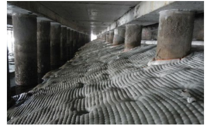
Figure 3. Mattress Under Deck
