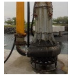
Figure 8. Dredging by Toyo Pump
