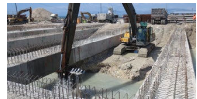
Figure 12. Excavator Working Between Beams
