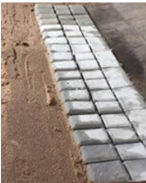
Figure 52. Test 5, As Constructed
