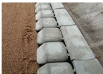
Figure 42. Test 1, As Constructed
