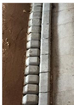
Figure 47. Test 3, As Constructed
