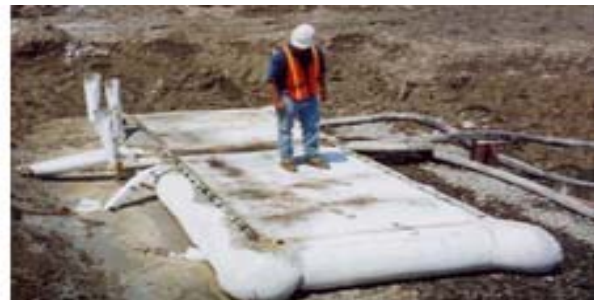
Figure 2: Grout Bag Trial
