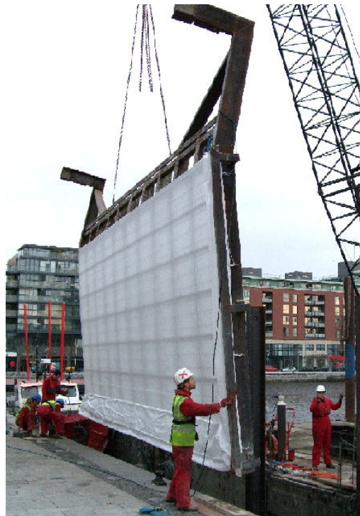
Figure 32: Fabric Formwork Facing Attached to Framework
