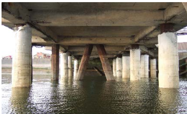
Figure 31: Dublin Pile Repairs
