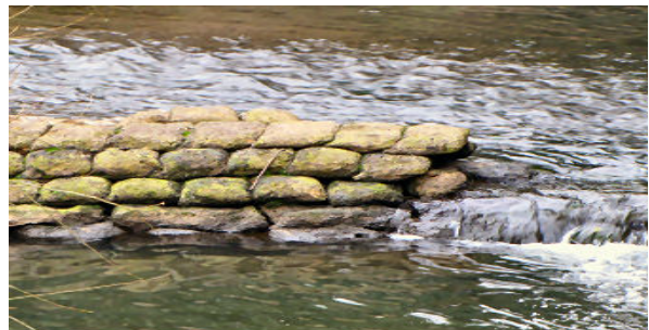
Figure 34: Concrete Bagwork
