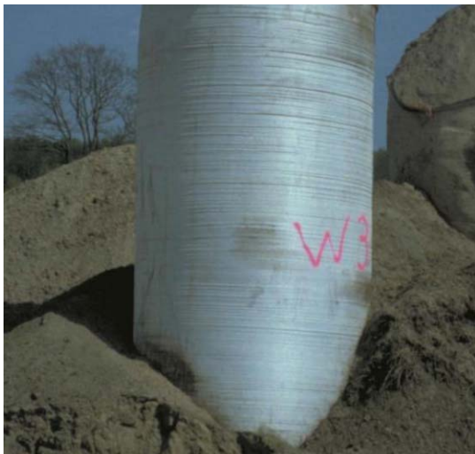
Figure 38: Pile Liner (Courtesy of Huesker)
