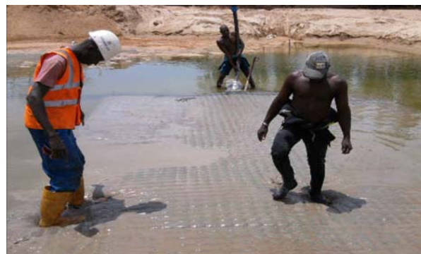
Figure 16: Mattress Trial Filling on Site
