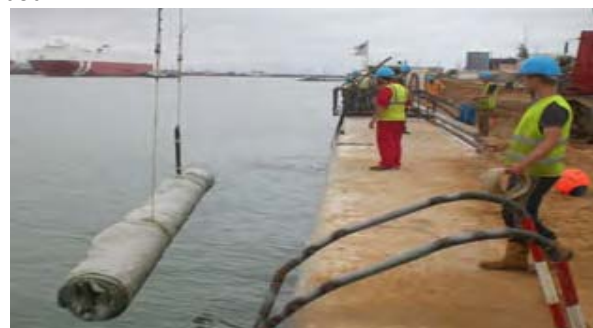
Figure 17: Lowering Mattress to be Rolled Out by Divers
