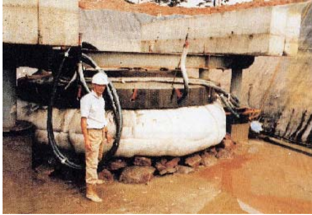
Figure 4: Grout Bag Trial Filling
