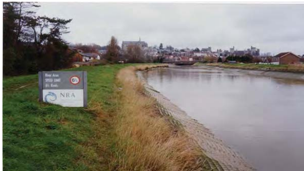
Figure 19: Mattress Revetment Currently
