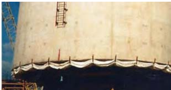
Figure 23: Seals Positioned with Break Ties
