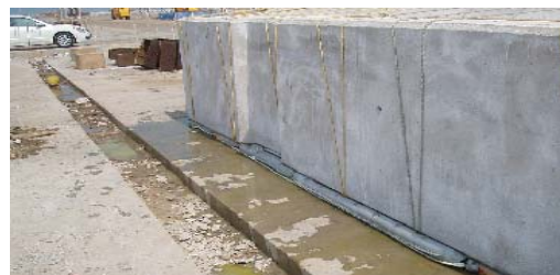
Figure 36: Grout Bag Bearing
