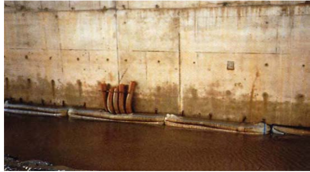
Figure 24: Filled Seals at Base of Caisson
