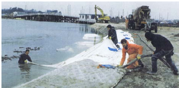
Figure 1: Concrete Mattress Installation
