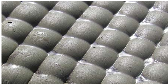
Figure 10: Filled Constant Thickness Mattress
