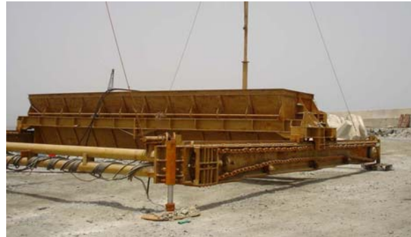
Figure 4—Traveling Screed Hopper (Khor Fakkan)
