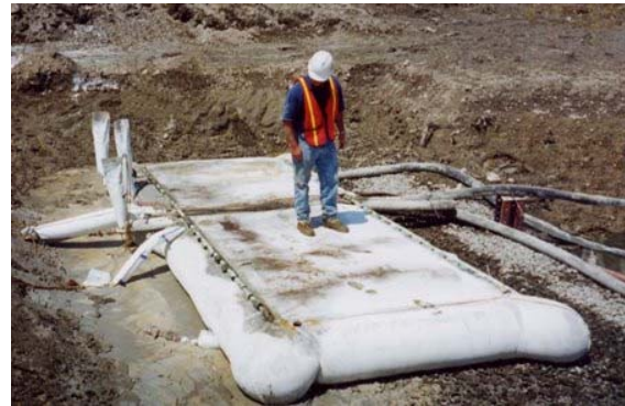
Figure 25 – Grout Bag Trials
