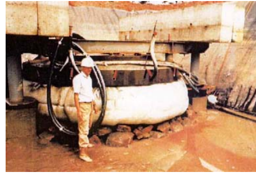
Figure 30 – Trial Forms Filled. P.E.I.
