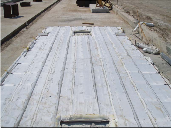
Fig 34, Grout Bag Shear Keys
