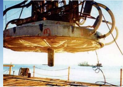
Figure 21 – Initial Pad, Forms Condensed
