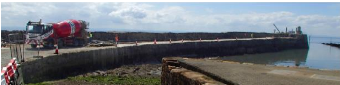
Figure 9 Concrete Pumping 270m
