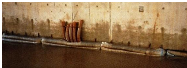
Figure 22 Concrete Grout Bags Foundations To Caissons, (Second Severn Crossing, UK)
