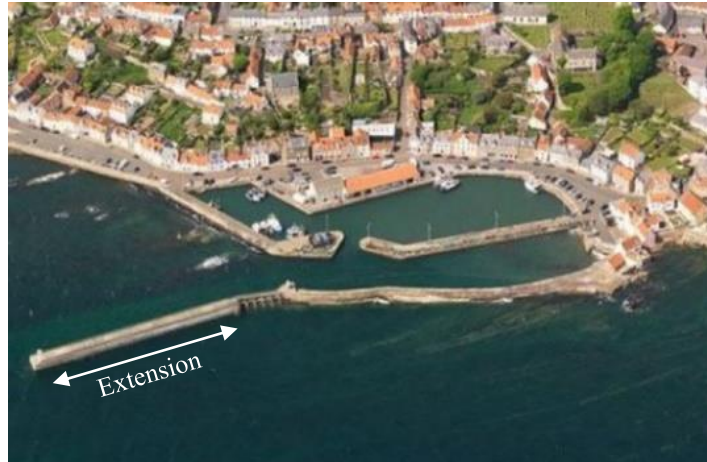
Figure 5 Pittenweem Breakwater Extension
