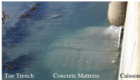
Figure 8 Picture Of Concrete Mattress (At Low Tide)
