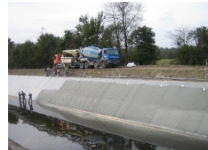
Figure 3: Concrete Mattress
