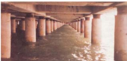
Fig. 2 – Pile Protection Mombasa
