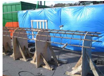
Fig. 5 – Reinforcement Cage
