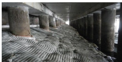
Figure 35. Open Hole Concrete Mattress, Puerto Quetzal, Guatemala
