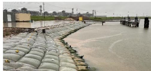
Figure 38. Open Hole Flex Mattress, Freeport, Texas
